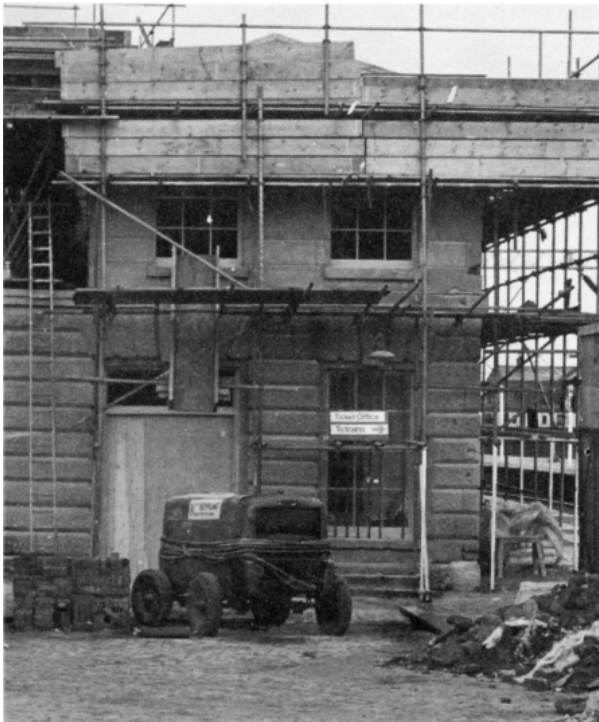
Rehabilitation in progress
