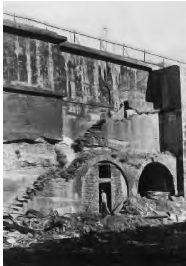
North side engineer's staircase, with boiler houses below
