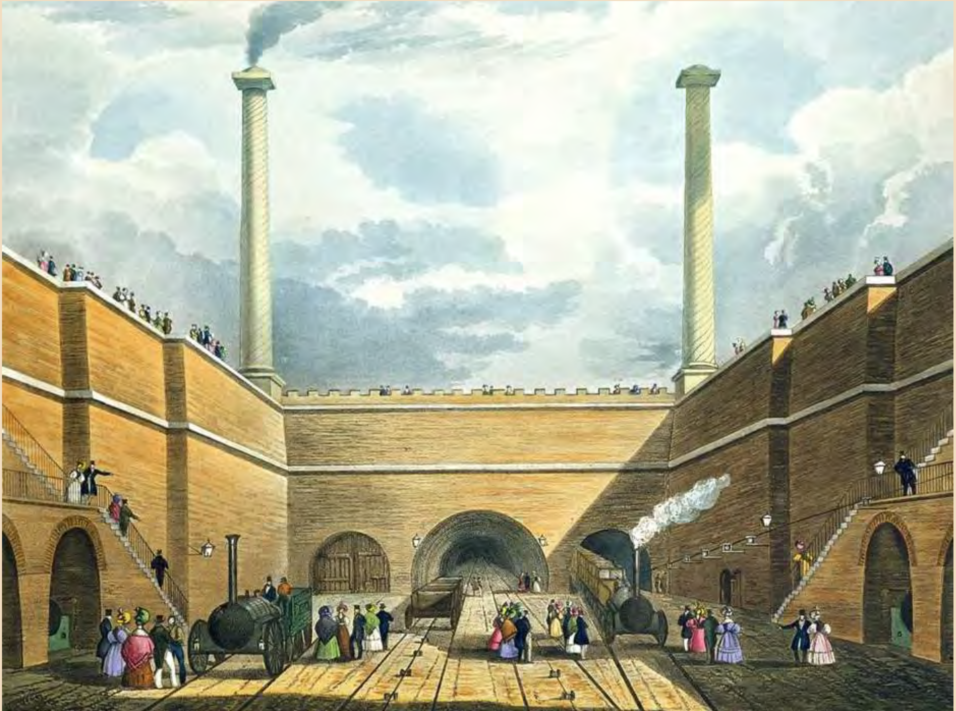
Entrance of the Railway at Edge Hill, Liverpool.
