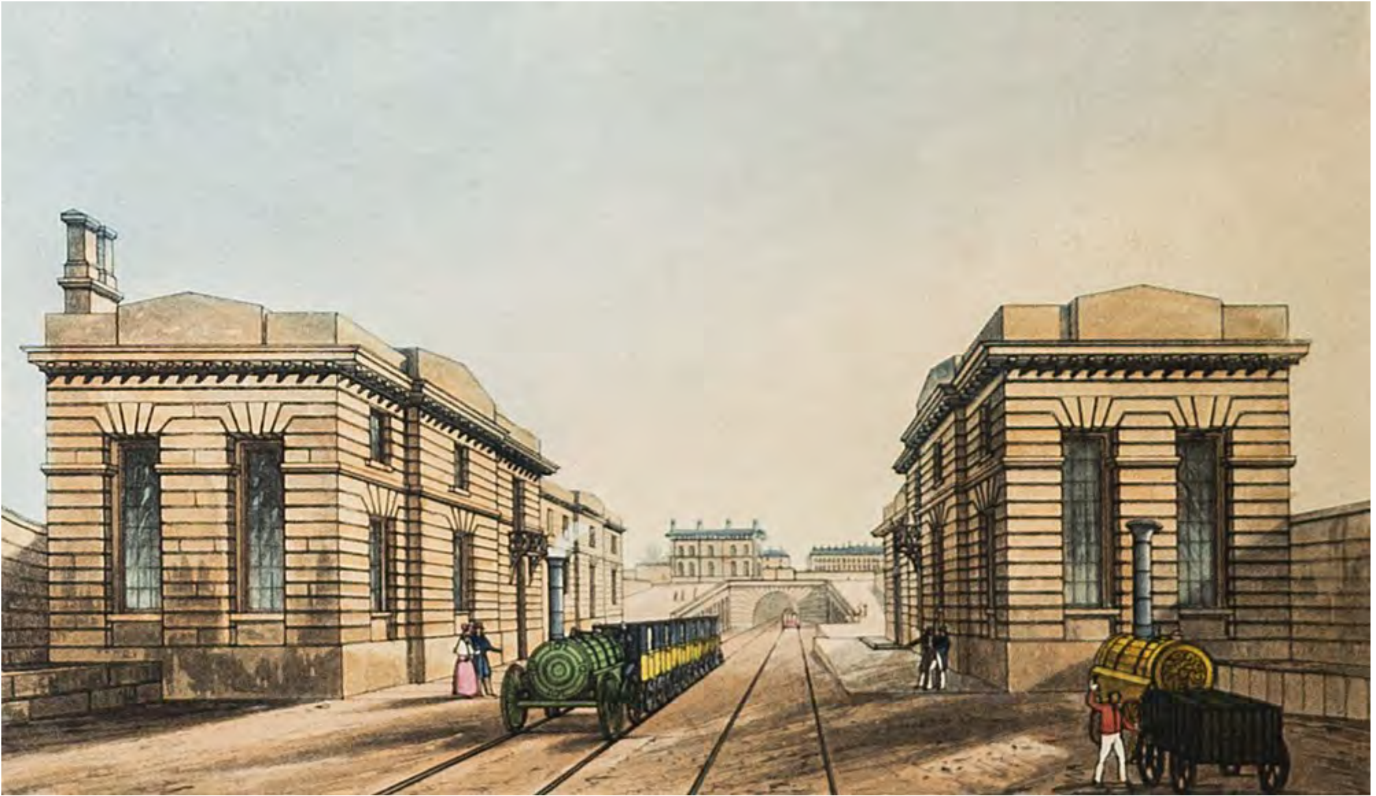
Edge Hill Station. End of tunnel. Ackermann & Co. (publ 1836)
