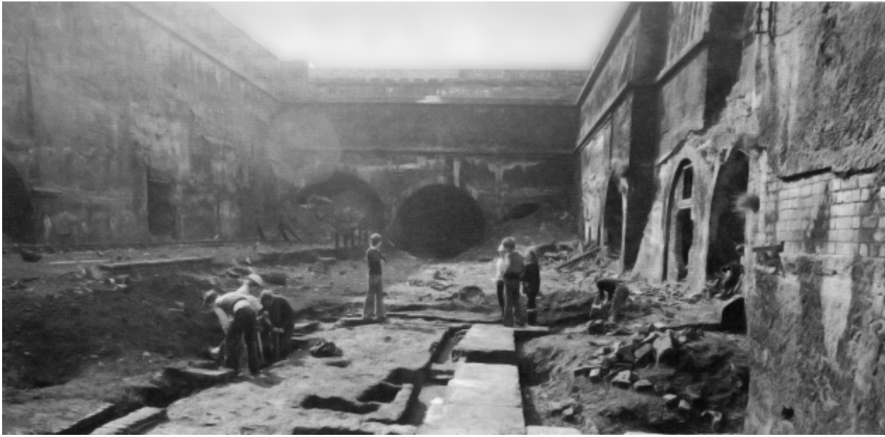
Foundations of the Moorish Arch under excavation, 1978.
