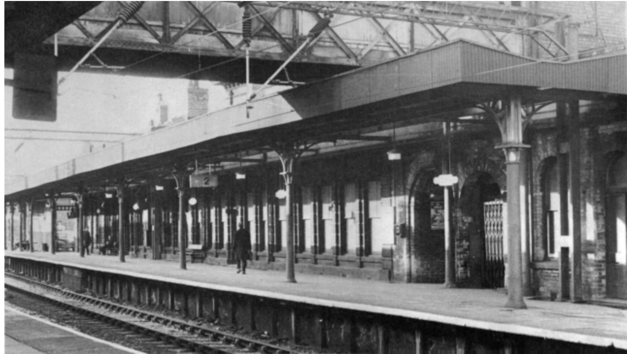
No. 2 platform just before demolition and rehabilitation
